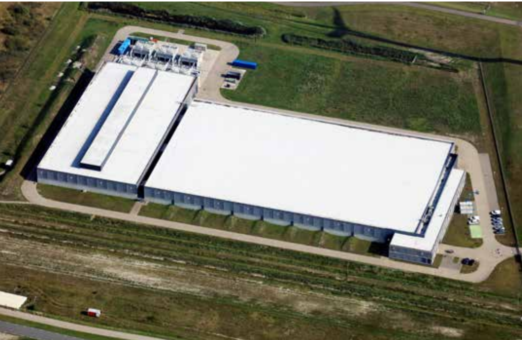
Datacenter QTS Eemshaven
