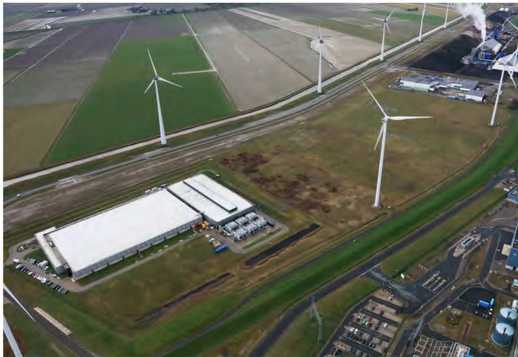
Datacenter QTS Eemshaven
