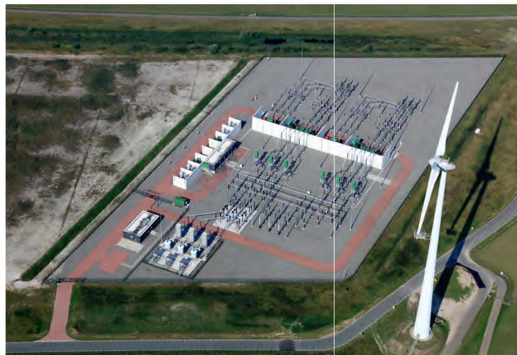
Transformatorstation Gemini Windpark Eemshaven
